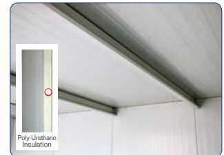
Building Reinforced with Metal Columns and Beams. ○ -Panel Walls are Fire-retardant CFC Free Poly-Urethane Insulation.
