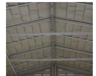
Strong Steel Roof Truss Carries 20 lbs/sqft Snow Load
