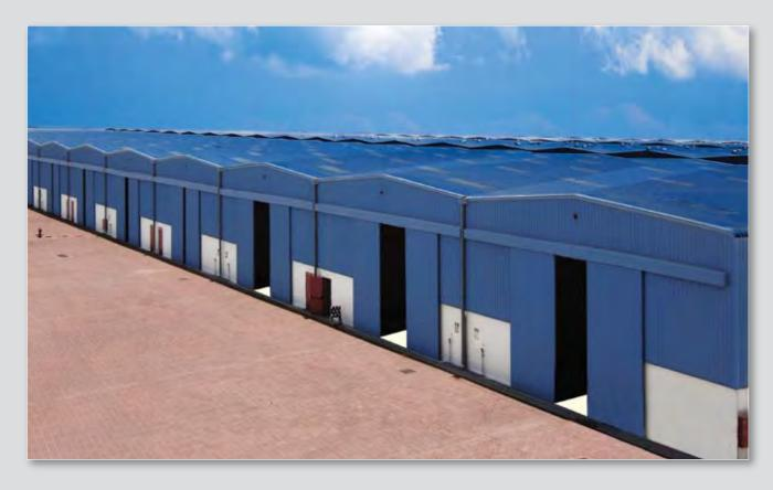
The complete system of pre-insulated monolithic composite panels manufactured by the Group offer excellent acoustic and thermal insulation for building roofs and walls for various kinds of industrial and civil structures.
